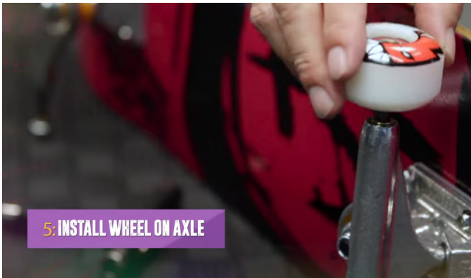
Step 5: Install the wheel onto the axle.
